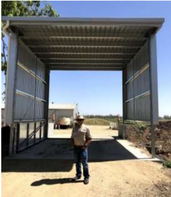
Figure 11. Newly-built truck wash equipment at entrance to Aus Sweetpotato Seed, Rockhampton
