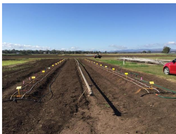
Plate 14. Plant bed irrigation system.
