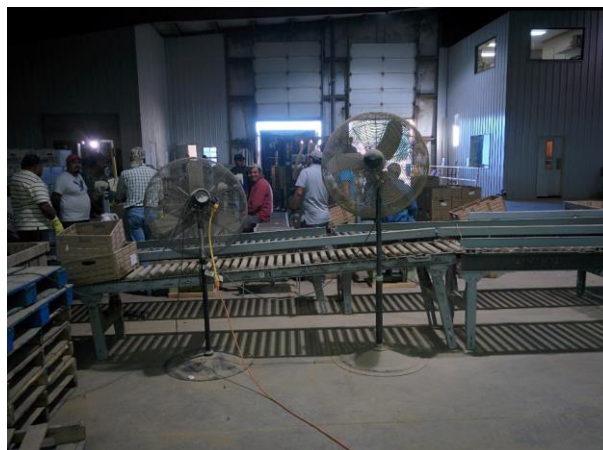
Plate 119. Large Louisiana packing shed.
